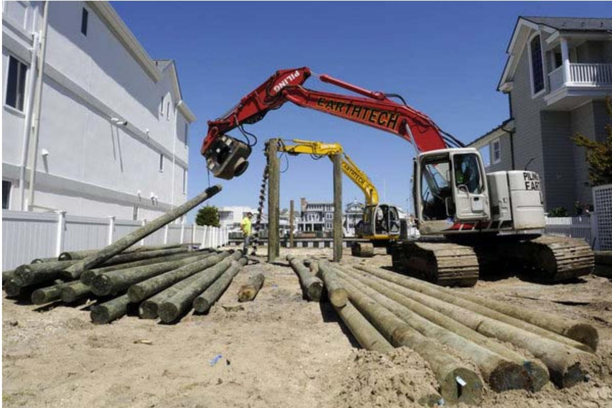
Workers from EarthTech of Ocean View, N.J., drive foundations at a homesite in Ocean City, N.J. Post-Sandy construction guidelines suggest pilings instead of blocks, even in flood zones that are not subject to the direct wave impact of a velocity zone. (TOM GRALISH / Staff Photographer)
